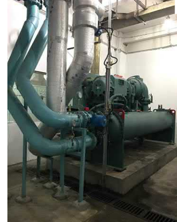
Air Conditioning Remodeling
