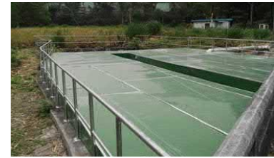
VOC-rich water storage tank
