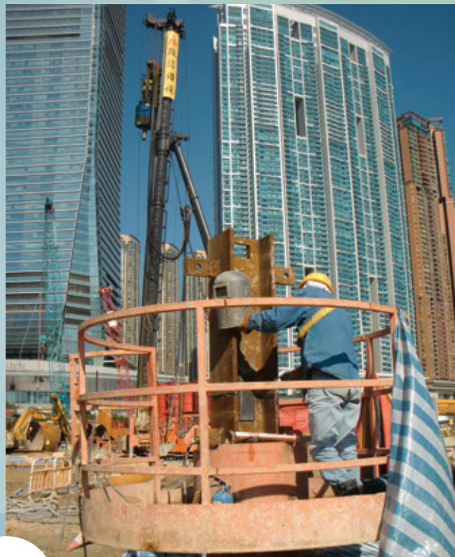
Welding for H-pile
